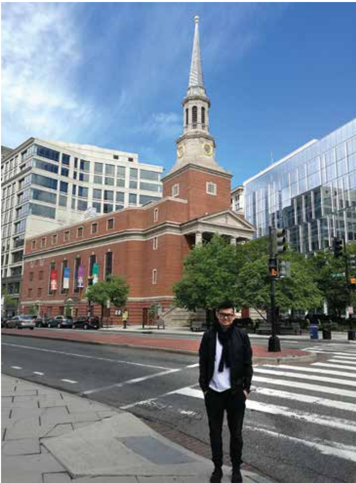
The New York Avenue Presbyterian Church.
